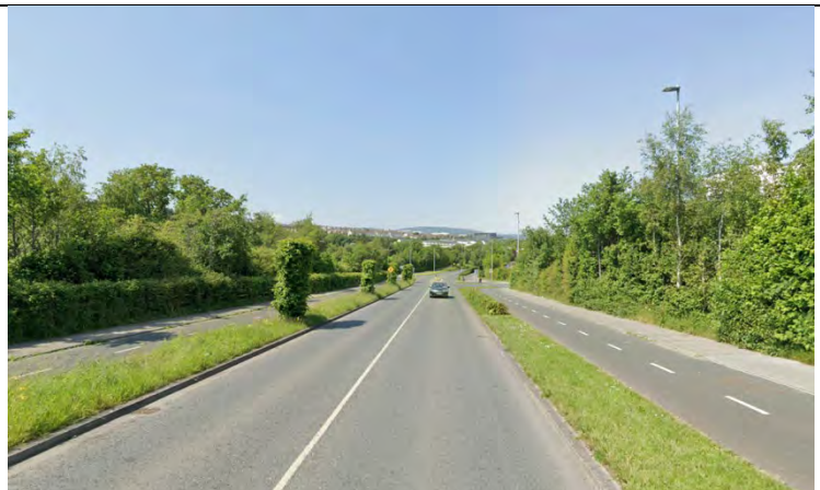
Port Access Road
